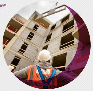
An i-SIP system provides a rigid composite building element with excellent stiffness, strength-to-weight ratio and durability. Complicated shapes and angles can be produced more economically and customised room shapes and sizes designed and installed without the need for additional costly frames or supports.
