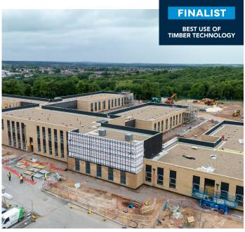
Designed by Arc Partnership and procured via the SCAPE Framework, Innovaré Offsite were appointed by main contractor Morgan Sindall Construction to design, engineer, manufacture and install our multi-award-winning i-FAST panelised system with the inclusion of factory fitted windows and external cladding for the new £30 million Horizons Academy, built on the former Ravensdale School site in Mansfield. The academy will support 160 pupils aged 7–19 with special educational needs (SEN)..
