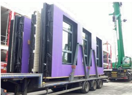
7 - Delivery to Site
